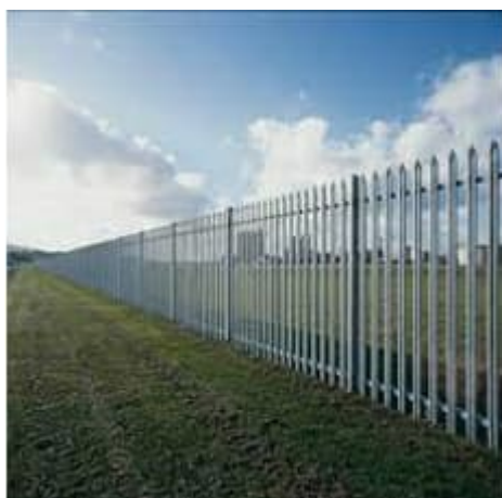
Plate 3-15. Standard palisade fencing
